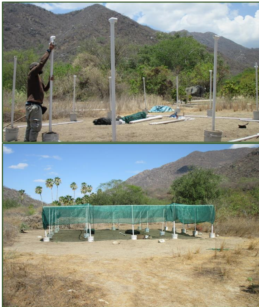
Construction and assembly of structures for the nursery in San Dionisio.
